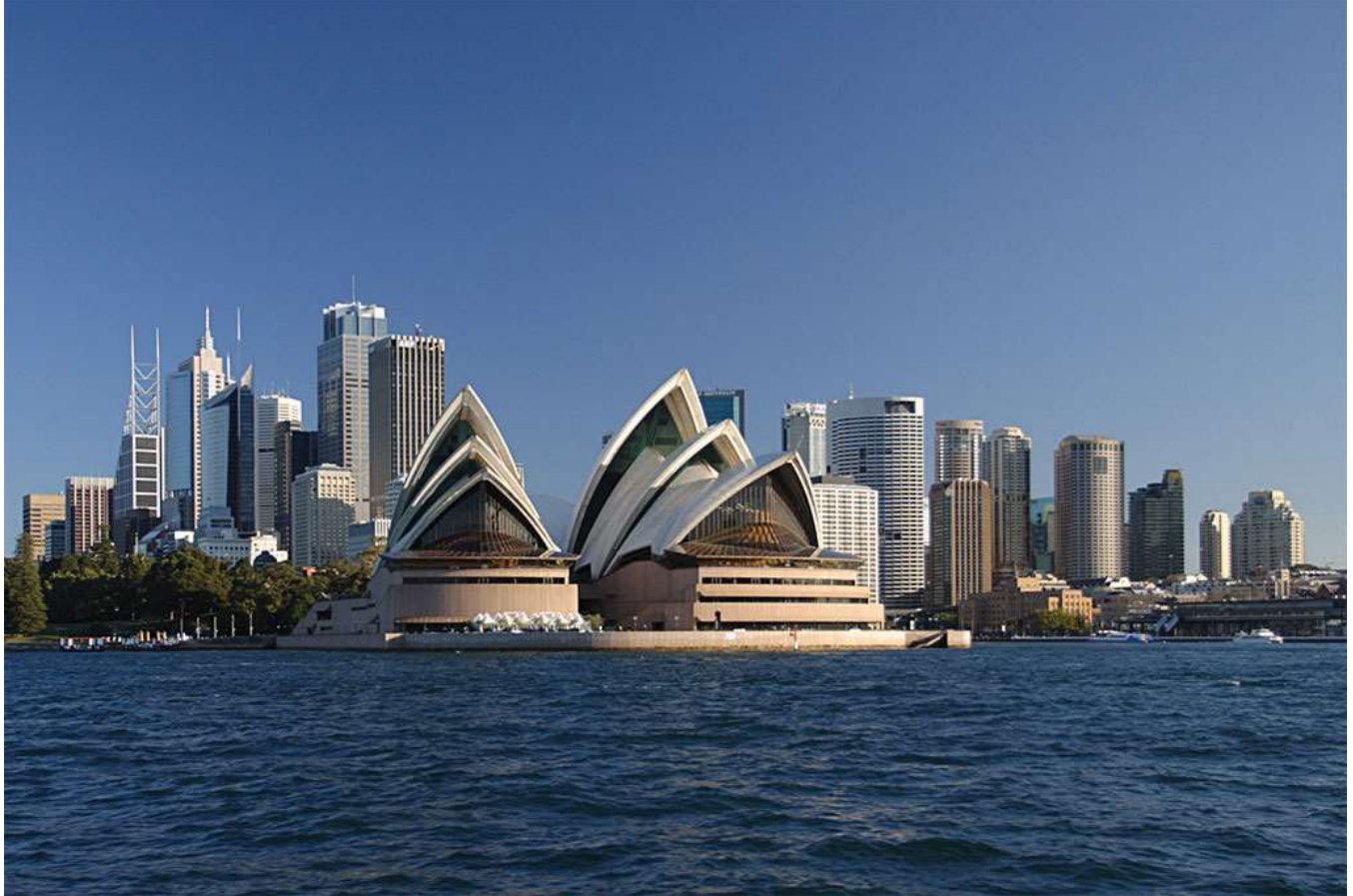
Figure 12.7 The Sydney Opera House Viewed from the Water with the City Skyline
